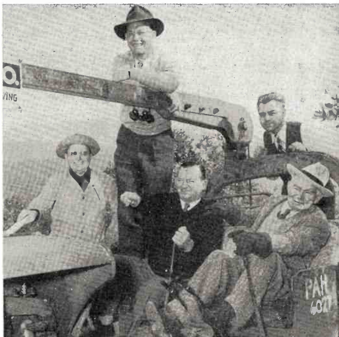
BREAKING GROUND for new KFI Los Angeles FM-television transmitters atop Mt. Wilson, Cal., this station executive-engineering group guided a bulldozer over the site during recent formal ceremonies staged in November. Structure to house FM transmitter will be erected at estimated cost of $100,000 and take nearly a year to build. Construction on television transmitter will not start until war's end. Bulldozer operators (1 to r, seated) are: William B. Ryan, general manager of KFI and Dr. Lee de Forest, pioneer scientist in radio and television; with supervisory engineering trio, H. L. Blatterman and Curtis Mason, station co-chief engineers; Seymour Johnson, consulting engineer.
